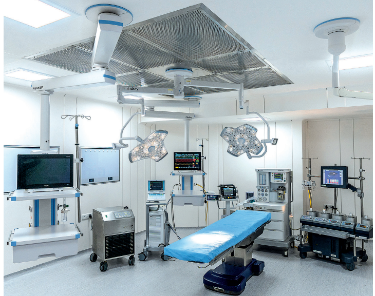
Cardiac OT with HEPA Filters & Laminar Flow
